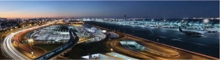
SurfaPaint ThermoDry Exterior for heat protection, Dubai Airport Freezone Area Warehouse.
